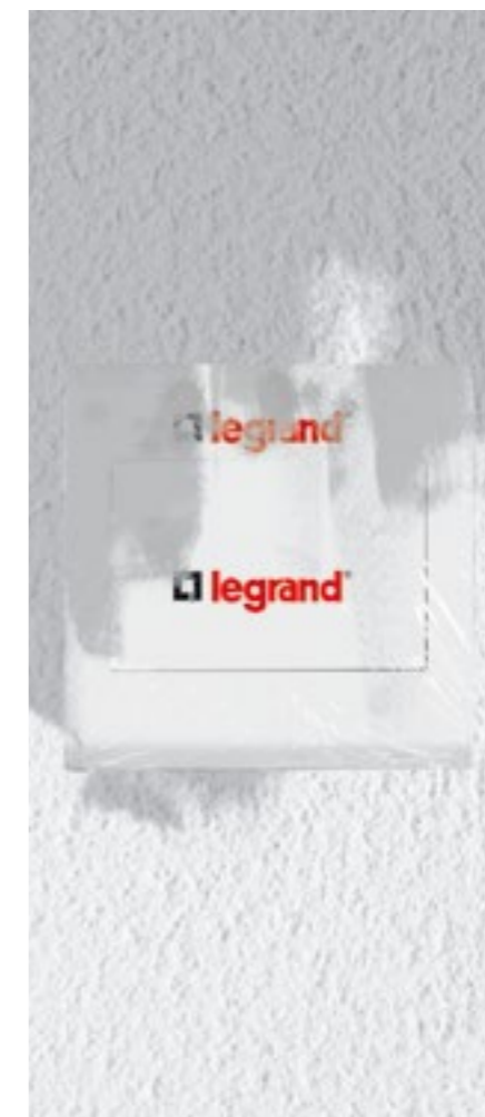
Only the soft protective film will get stained by the ongoing wall paintwork.
